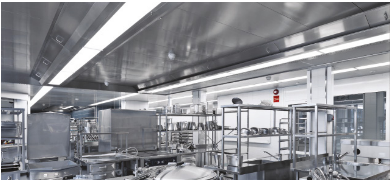
Kotka central kitchen (Kotka, Finland)
